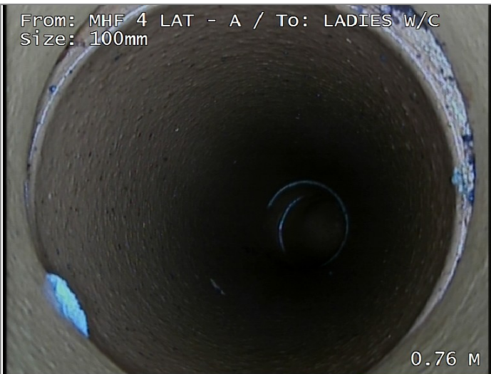
Joint displaced medium - Remark: TISSUE CATCHING
