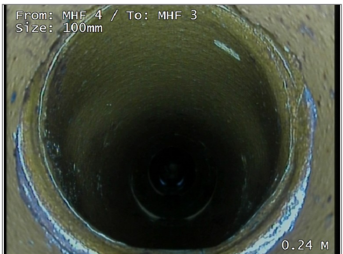
Joint displaced medium
