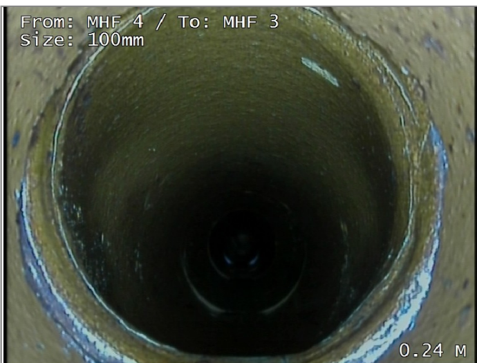
Cracks multiple from 12 to 12 o'clock
