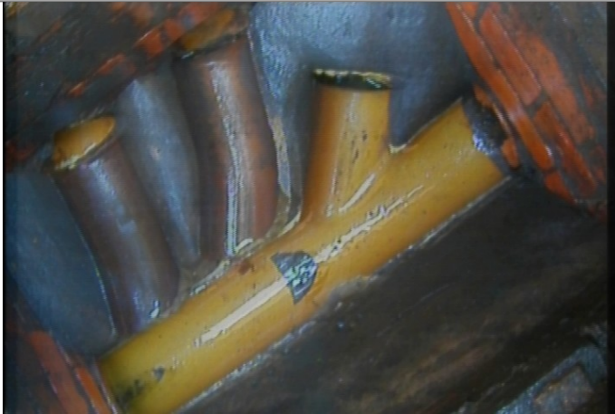
Manhole / Access Point: MHF 4 Internal
