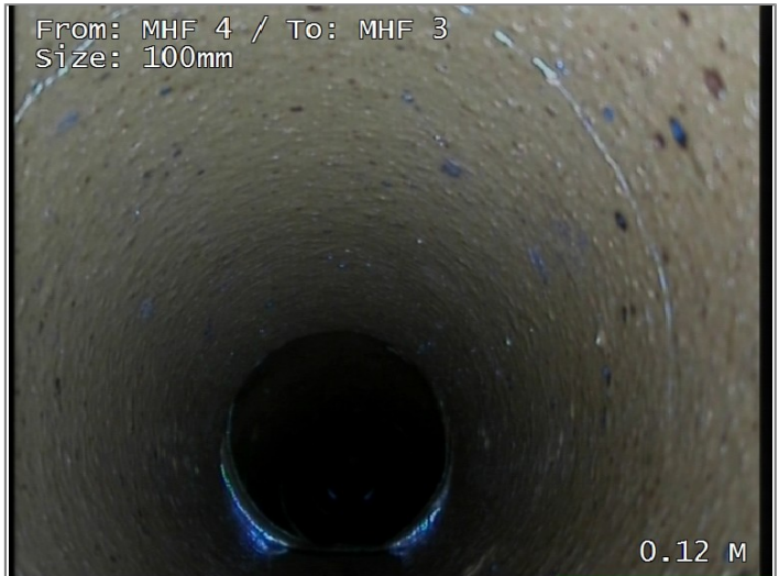
Crack circumferential from 12 to 12 o'clock
