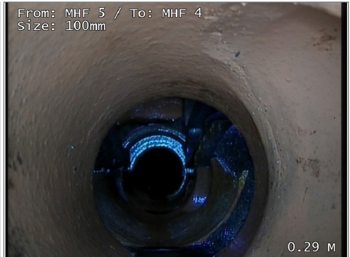
Junction at 3 o'clock, diameter 100mm - Remark: JUNCTION FOR GENTS W/C
