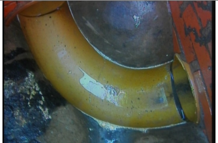
Manhole / Access Point: MHF 3 Internal
