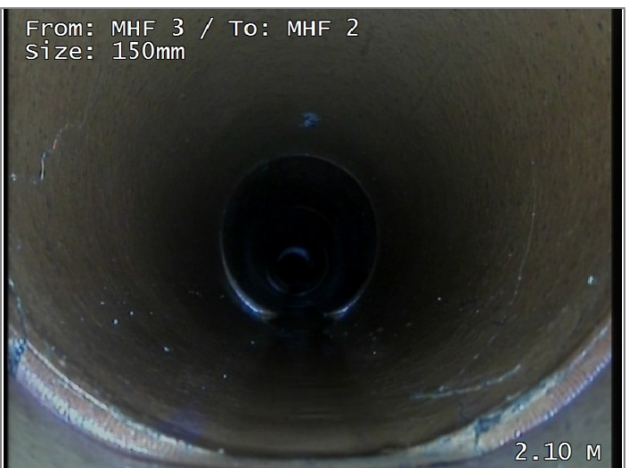
Cracks multiple from 12 to 12 o'clock
