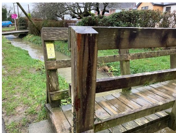
Photo 8: Upper section foot bridge alongside Manthrig Lane.
